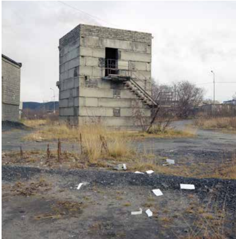
There are towers everywhere in Nikel. This one is about five metres tall, with iron stairs leading to a door. It's a waste depot of a type that is only found in Nikel. The hills of black sand in the background are from the smelter.
