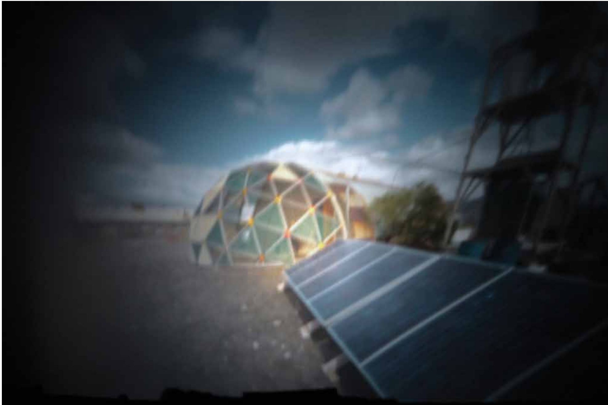
Clean Livin' 'South Base' (designed by JIMPARCH), Center for Land Use Interpretation, Wendover, Utah, 2009.
